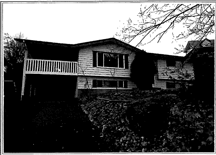
FRONT VIEW OF SUBJECT PROPERTY
