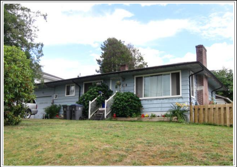
FRONT VIEW OF SUBJECT PROPERTY
