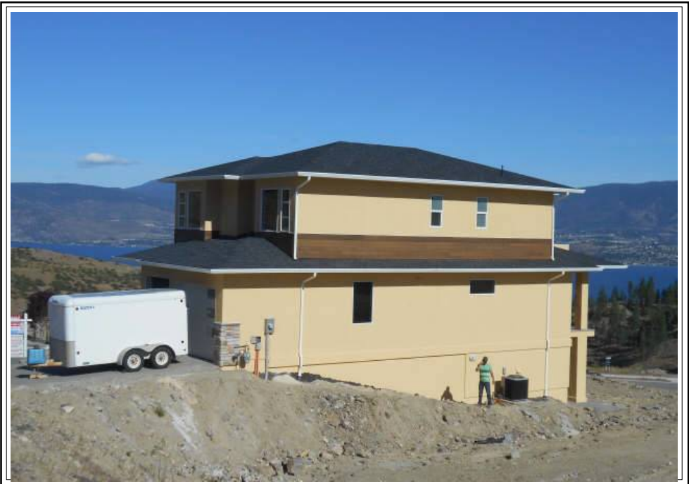
Side view of the house - Landscaping to be completed - finishing retaining walls, lawn irrigation and final landscaping and shrubbery.
