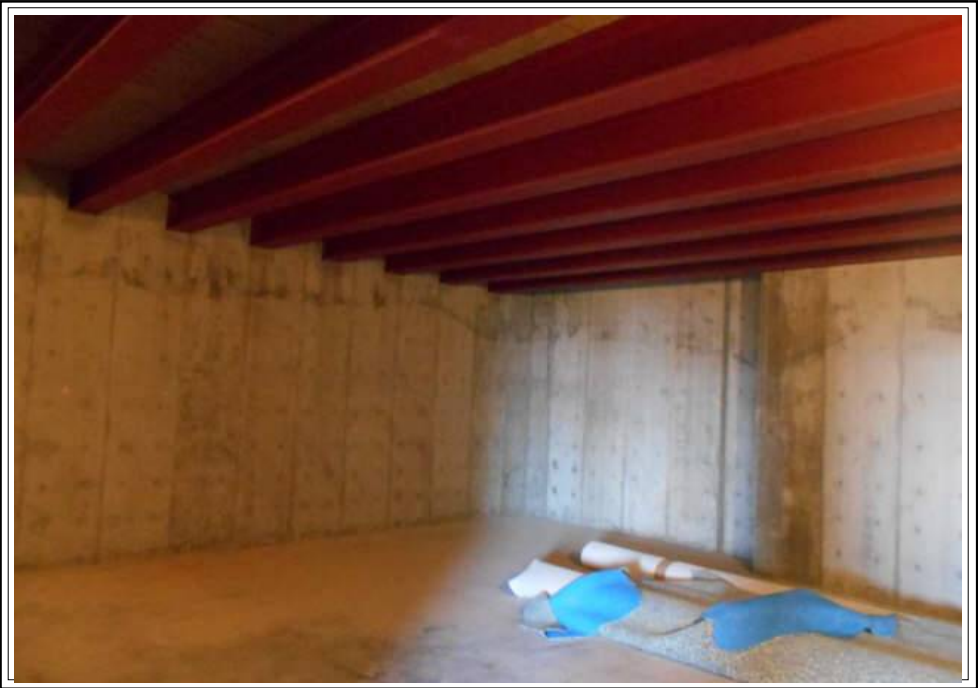
Basement - area below the garage Future media room - suspended slab
