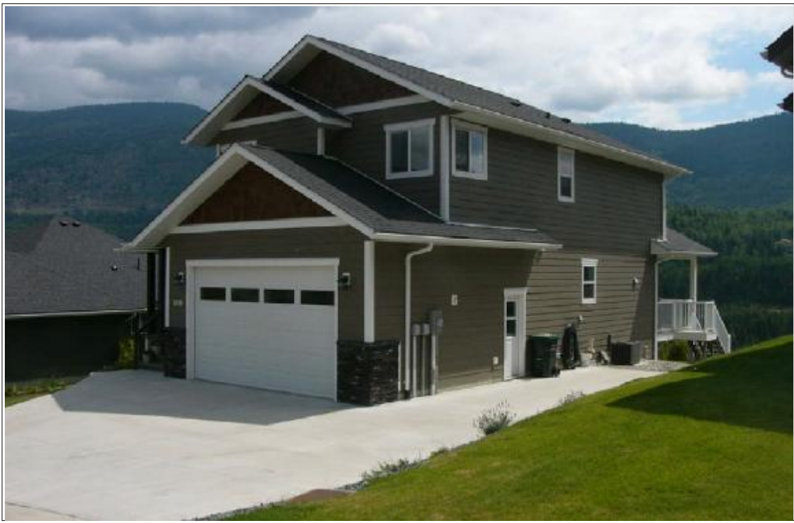
Front Elevation of Subject Property
